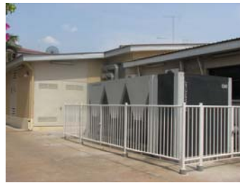
Construction of technical facilities of BSL3 (DBD) and Installation of cold group (CIAT/Comin Khmere)
