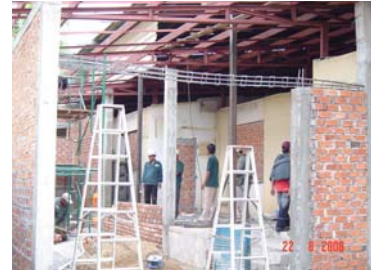
Heightening of the steel frame and the roof for the passage of the service shafts (DBD, Cambodia)
